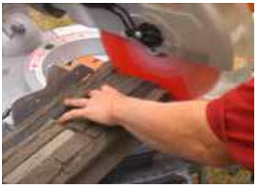
5. Cut panel with hand saw or table saw.
