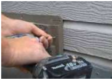
6. Screw or nail on side of panel for flash finish.
