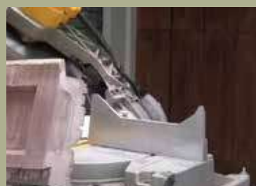
5. Cut panel with hand saw or table saw.
