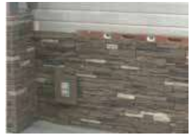
4. Check level during install.
