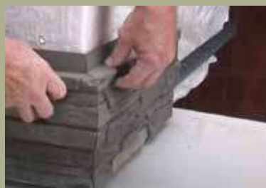
6. Screw or nail on side of panel for flash finish.
